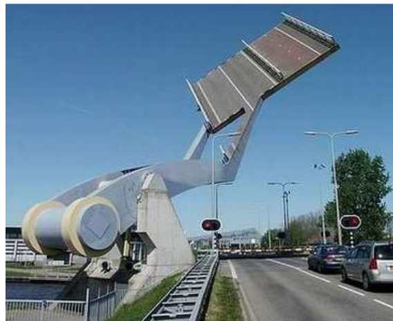
Figure 1. The Slauerhoff Bridge [7].
